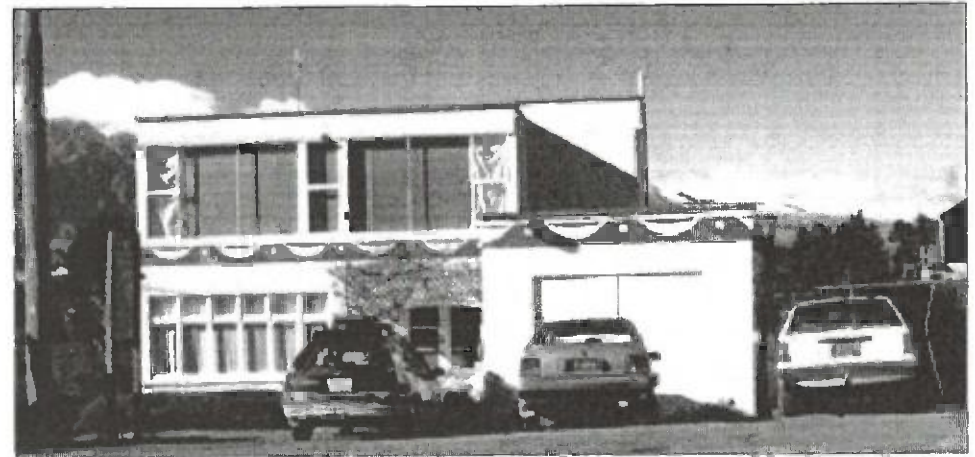
Man Street art deco, built in the late 50s by Eric Scheib, plasterer and general character. Demolished earlier this year to make way for car parking.
